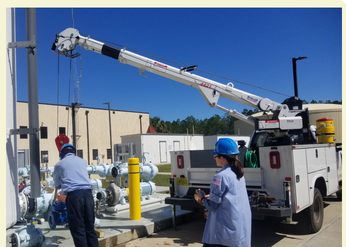
Filtrate Check Valve Replacements
