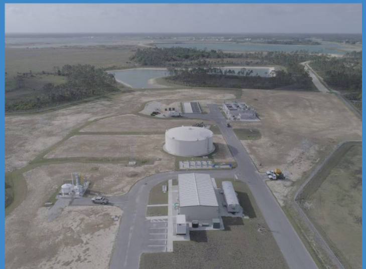
Babcock Ranch Water Treatment Facility
