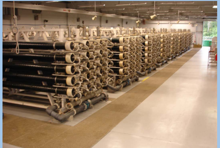
Southwest RO Plant 2 Addition Built in 1985
