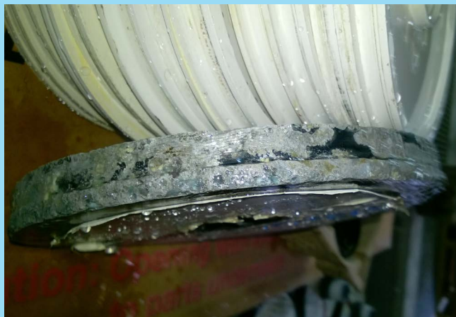
Eroded End Cap
