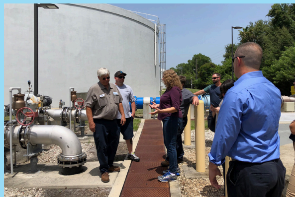
City of Clearwater Plant Tour
