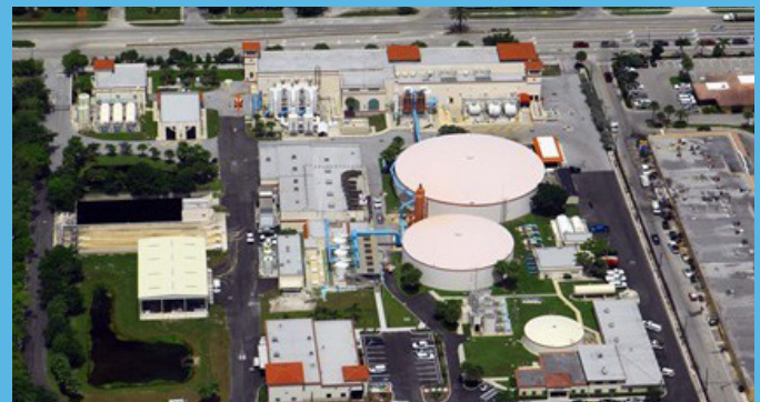
Jupiter Water Treatment Plant
