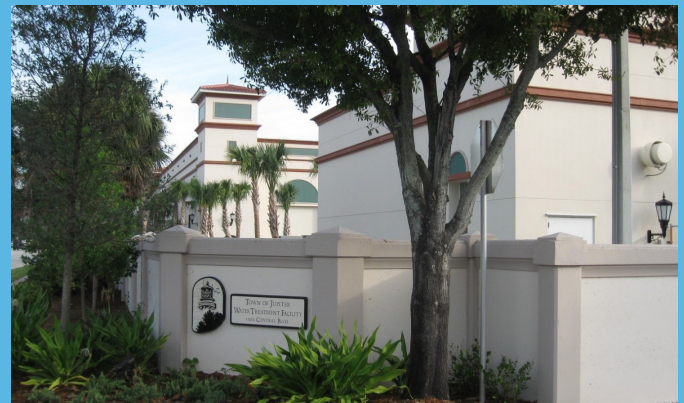
Jupiter Water Treatment Plant
