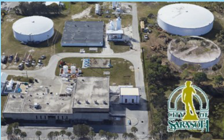
Figure 1: City of Sarasota Drinking Water Treatment Facility
