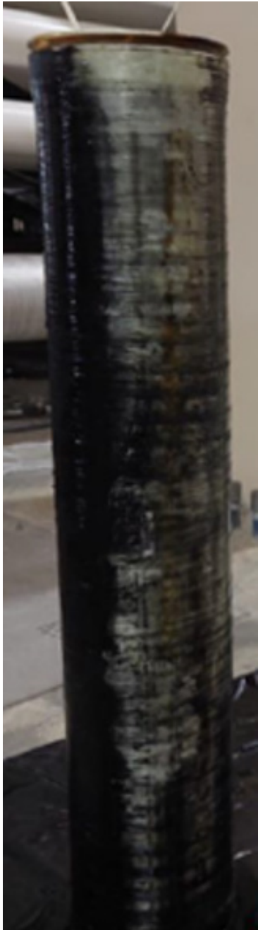
After membrane removal
